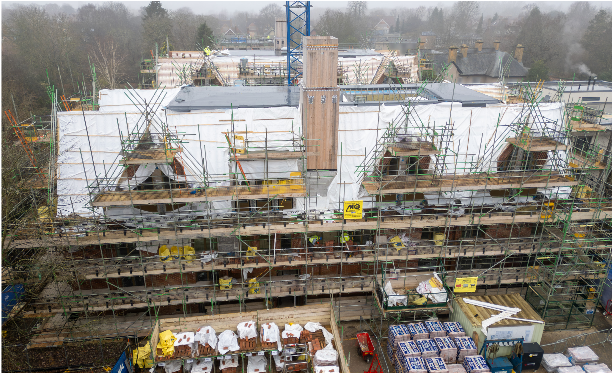
Dec 2024 – Waterproof membranes had been laid onto the roof of Water Court East in preparation for the roof battens and tiles to be laid.
