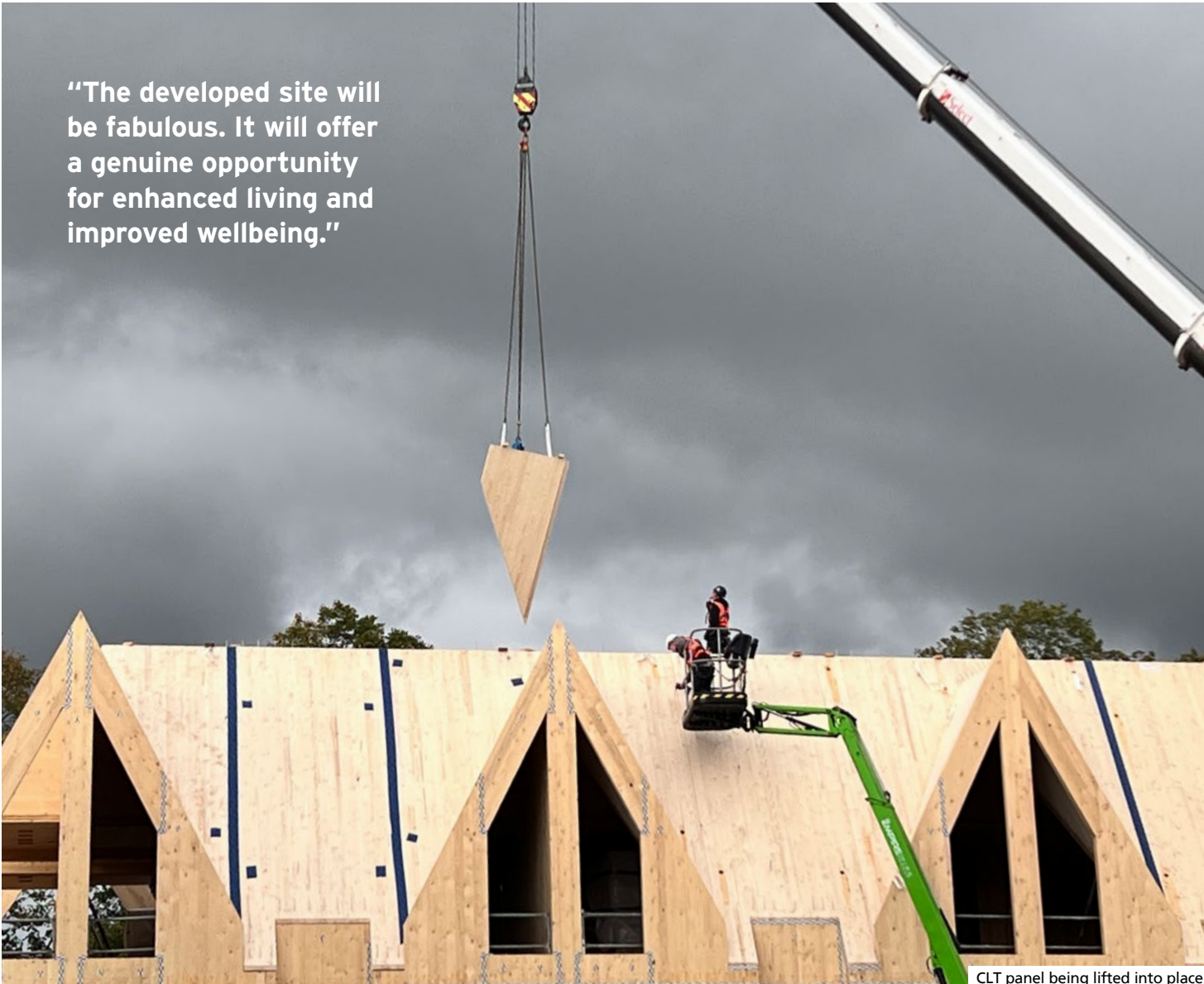
CLT panel being lifted into place
