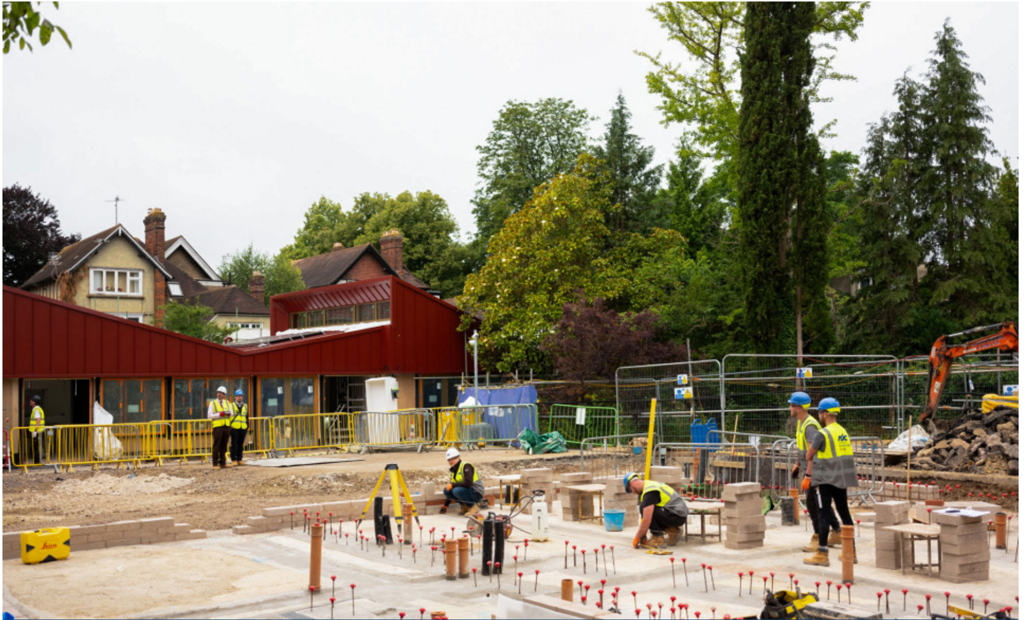
The blockwork for Woodstock Pavilion at an early stage.
