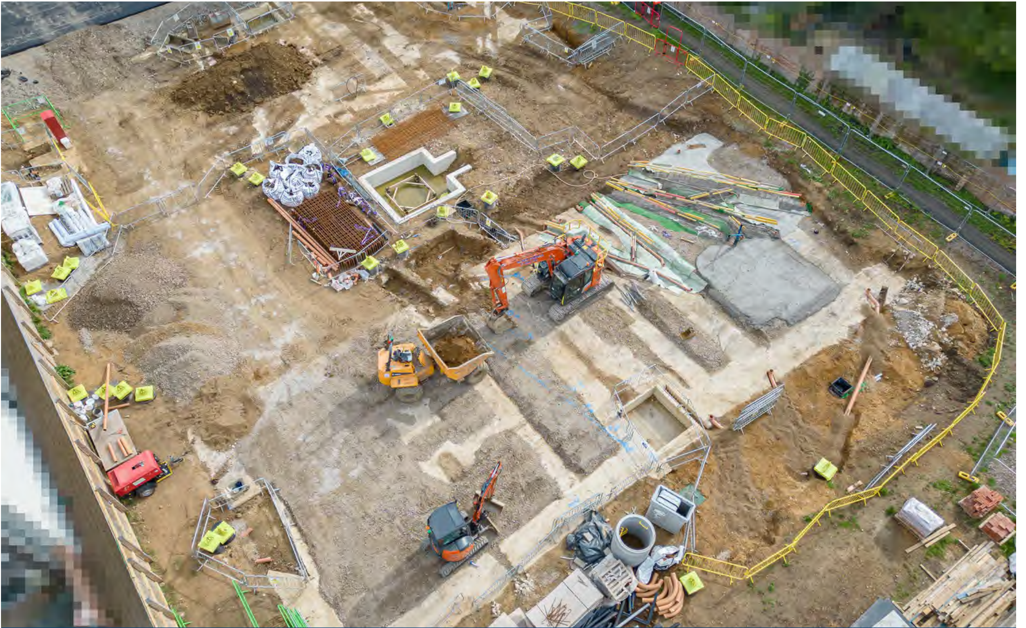
Image showing the foundations to Water Court West & Water Court East
