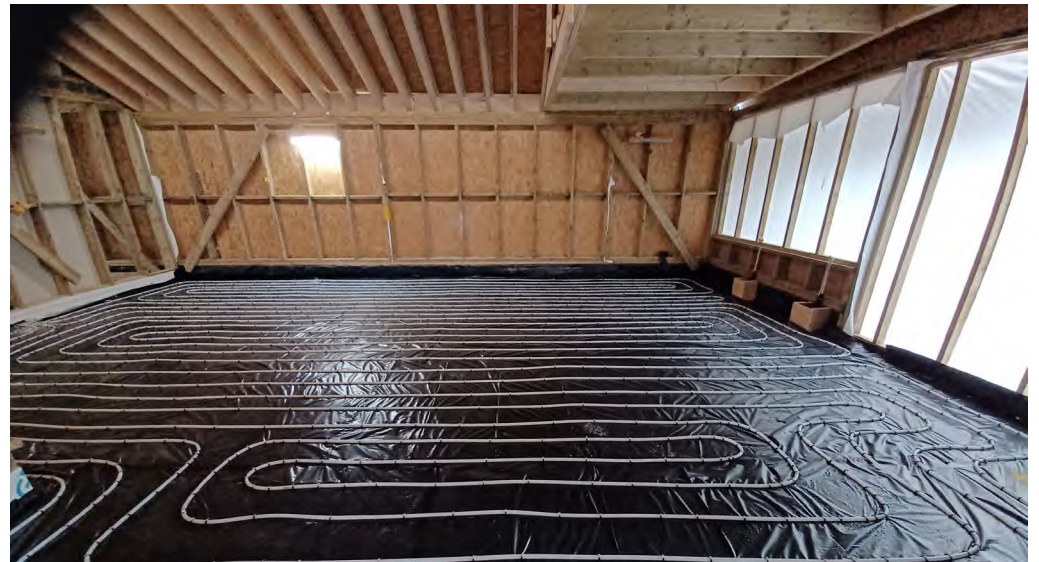
3-5 years room with underfloor heating pipework laid.
