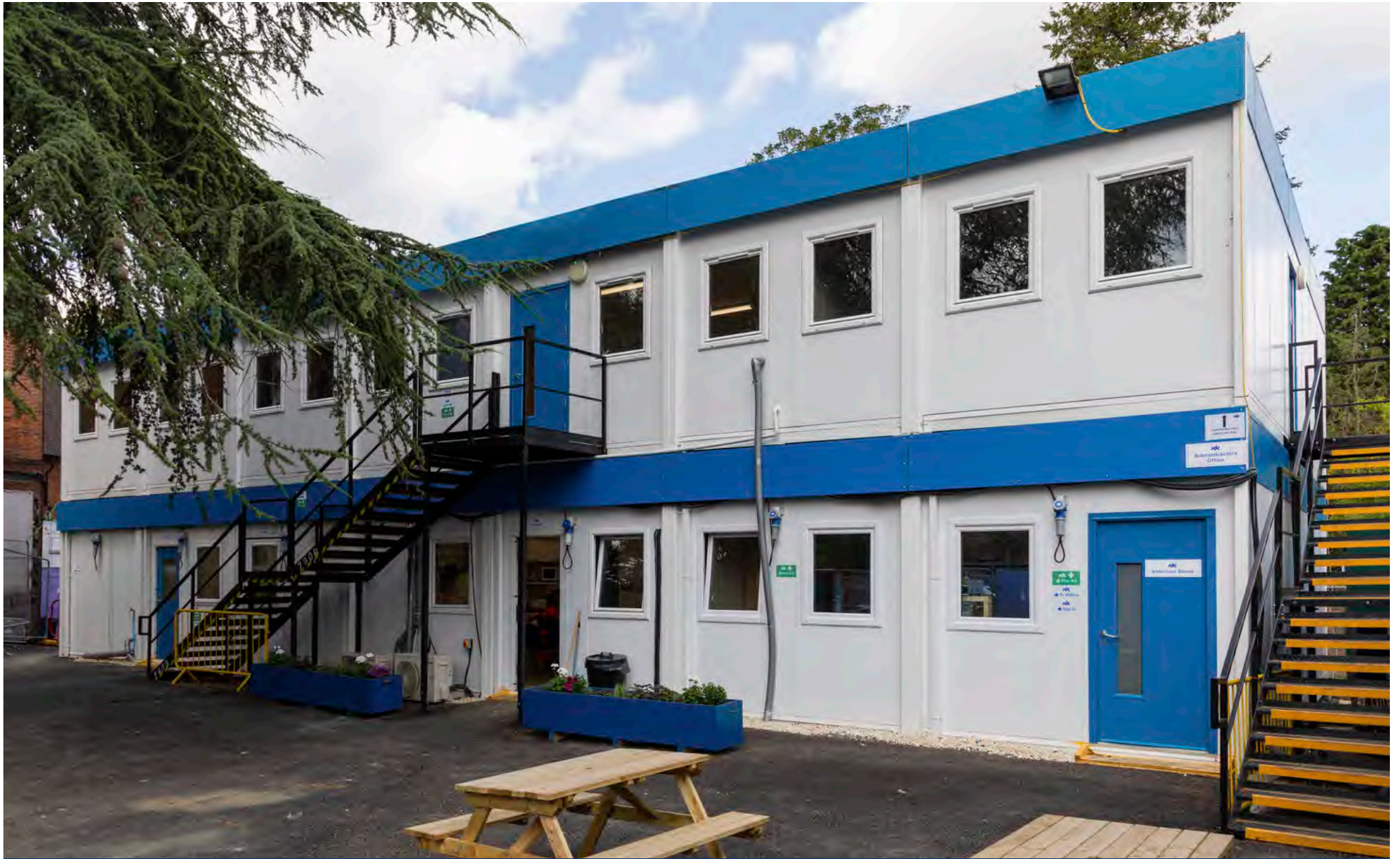
The site welfare units were assembled in spring 2023 for the project team to occupy. The facilities, include site offices, canteen, toilets, a drying/ changing room and prayer room.
