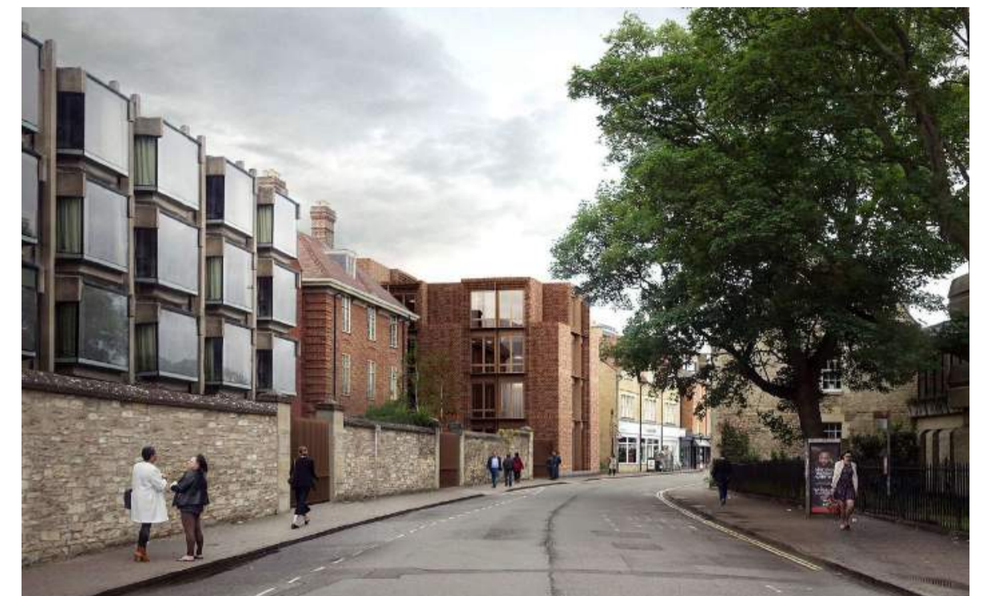
Catherine Hughes Project, Somerville College by NMLA. This building is CLT frame with a brick façade.
