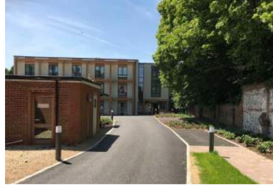
Fairfield Residential Home access - Cluttered approach from Banbury Road
